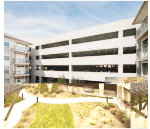
Pictured above left: The building form largely conceals a 500+ space parking garage. Above right: Open air decks reduced fire sprinkler and ventilation requirements.
