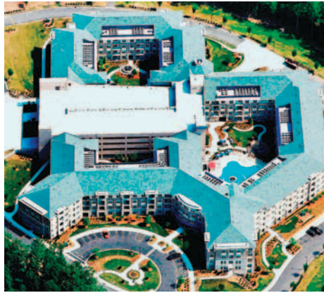
Pictured above left: The building form largely conceals a 500+ space parking garage. Above right: Open air decks reduced fire sprinkler and ventilation requirements.
